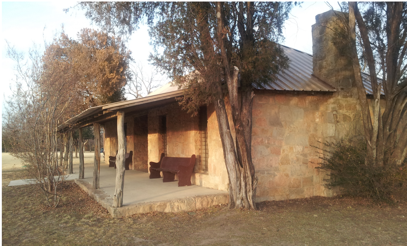
CAMP COLORADO REPLICA ADMINISTRATION BUILDING
